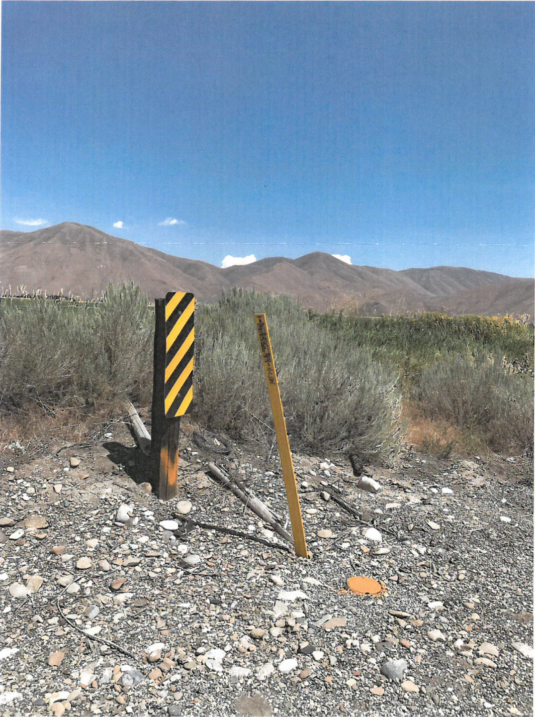
Figure 1: Line Marker Near Reg Station 50109
